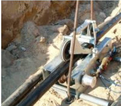
BKS 400 in a trench
