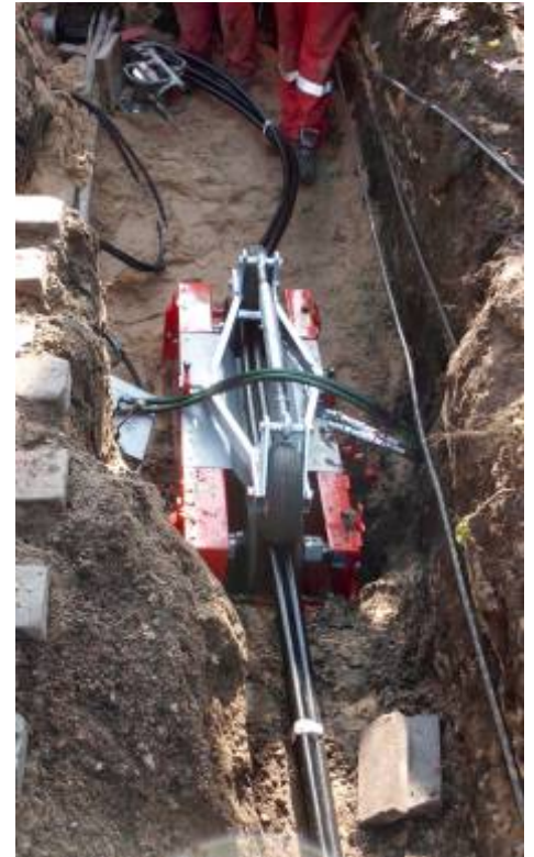
Laying of 3 x single core 30 kV
